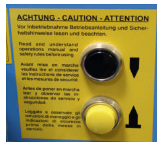
Fig. 33: Manually operated valve
